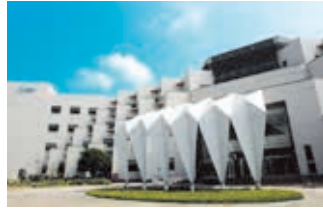
Tainan Plant (Diamond-rated Green Building)
