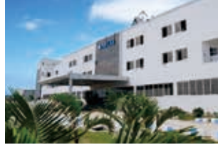
Rudrapur Plant (Green Building)
