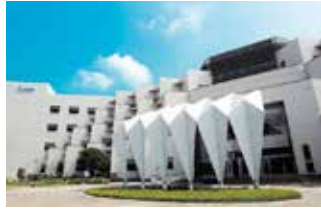
Tainan Plant (Diamond-rated Green Building)
