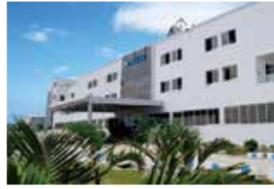
Rudrapur Plant (Green Building)
