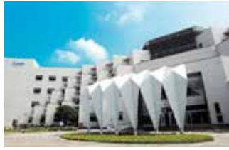
Tainan Plant (Diamond-rated Green Building)
