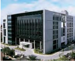
Taoyuan Technology Center (Green Building)
