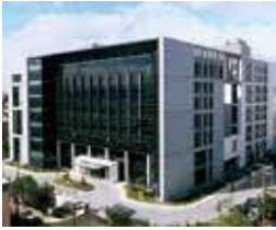
Таюан Technology Center (Green Building)
