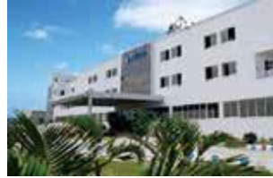
Rudrapur Plant (Green Building)
