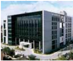
Taoyuan Technology Center (Green Building)
