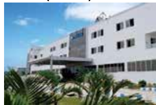
Rudrapur Plant (Green Building)
