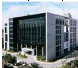
Taoyuan Technology Center (Green Building)
