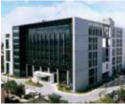
Taoyuan Technology Center (Green Building)
