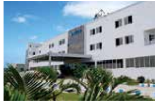
Rudrapur Plant (Green Building)
